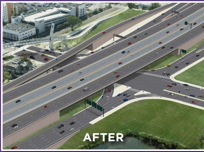
The current I-4/Colonial Drive restricts movements and traffic capacity. By replacing the loop ramps from westbound Colonial Drive to westbound I-4 and eastbound Colonial Drive to eastbound I-4 it will provide more direct access to I-4. By reconfiguring the interchange to a single-point urban interchange (SPUI) it will accommodate more vehicles.
