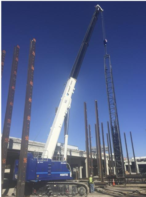
Two 130-ton capacity Tadano Mantis GTC-1200 cranes are a part of SGL Constructors' crawler crane fleet that are being utilized for pile driving and lifting work on the I-4 Ultimate project in Orlando.
