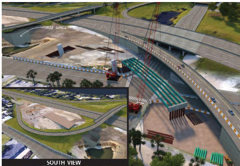
Artist rendition of steel girders placed above the Division Avenue and Gore Street intersection.
