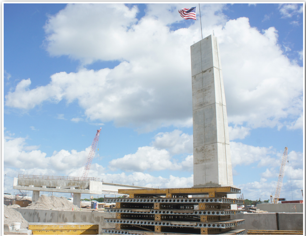
The first direct connect pylon is constructed near Lake Ivanhoe.
