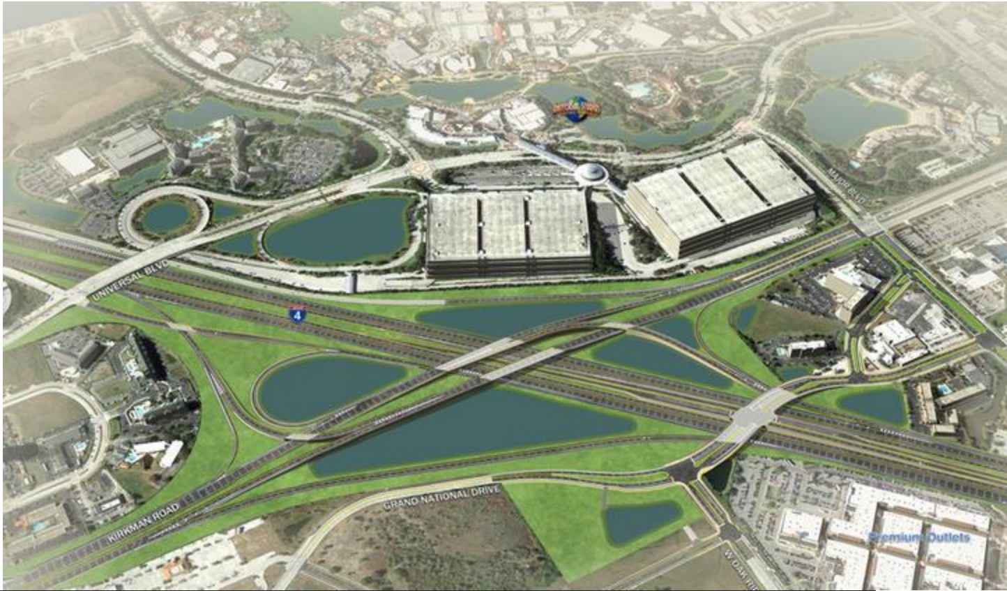
CAPTION I-4 Ultimate: I-4 and Kirkman Rd.
