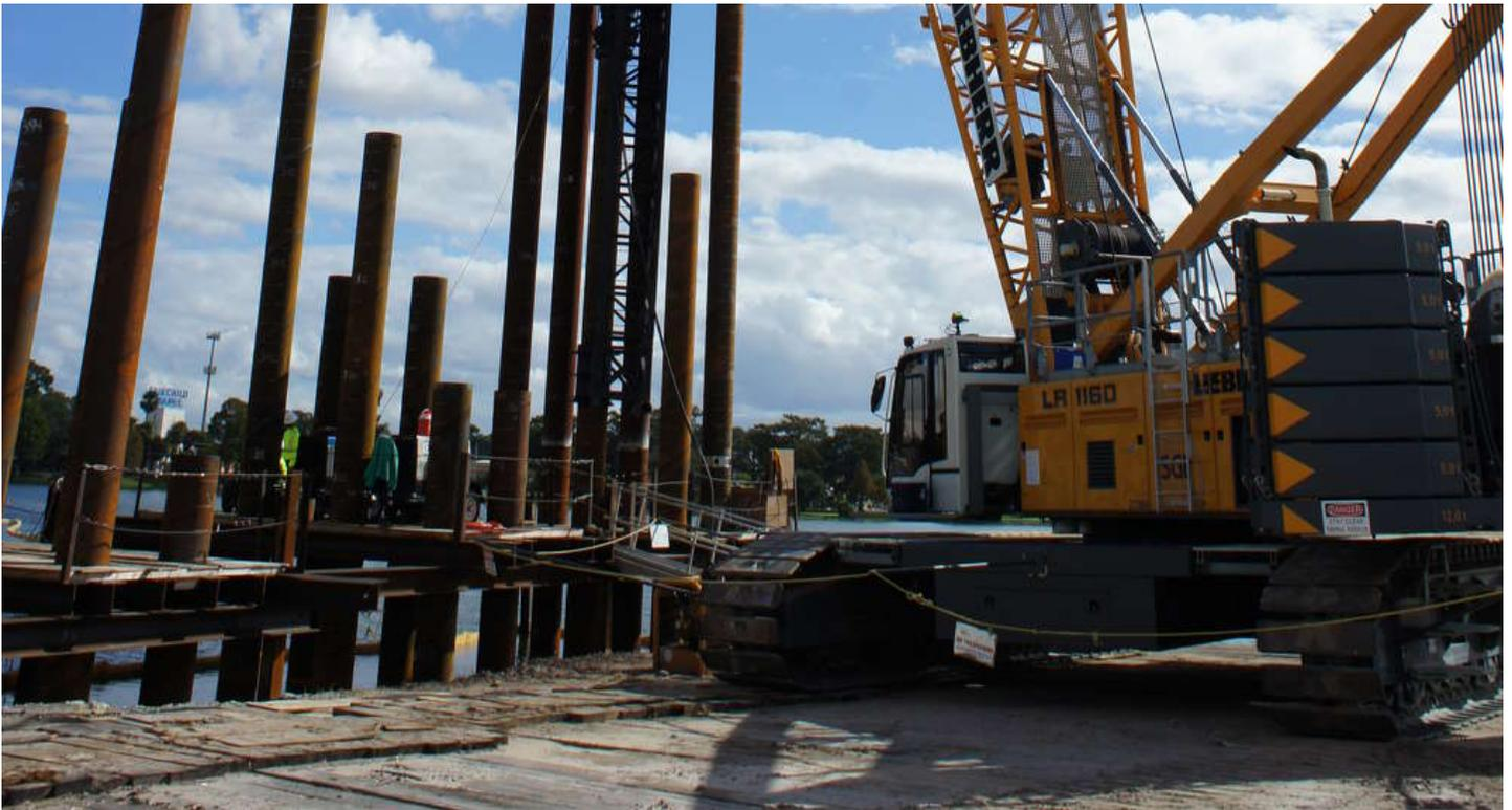
**FDOT? photo “The large Liebherr crawler cranes can be seen at almost every interchange, and are being used for pile driving and structure work when the work space allows,” said Jon Walker, SGL program project manager.**
